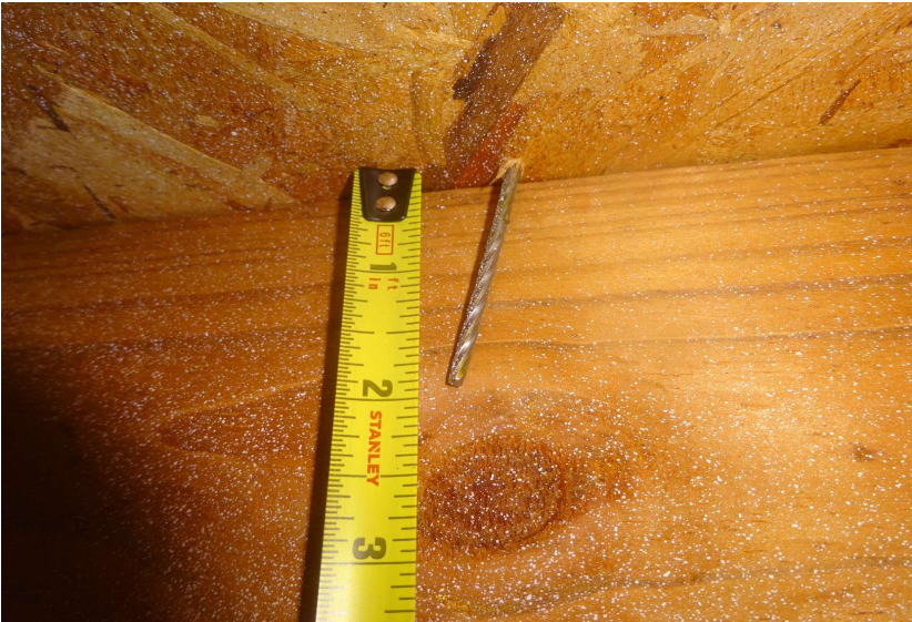
8d nails verified
